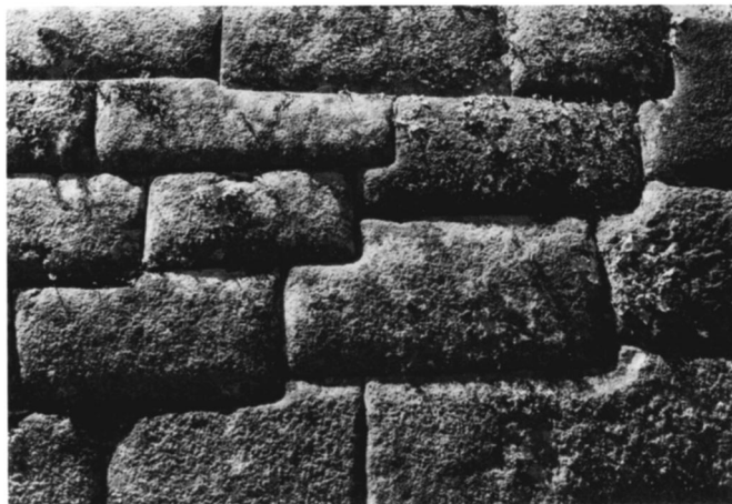
FIGURE 8: Akapana, Tiahuanaco: random-range work of small stones between large blocks on the west side
