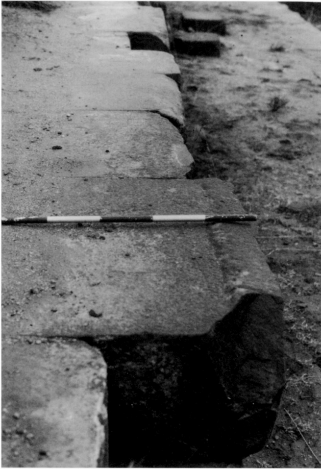
FIGURE 24: Pumapunku, Tiahuanaco: second terrace wall on south side showing a residual bulge
